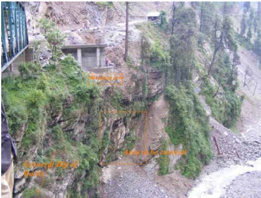
Picture 2 Site showing spot needing grouting and concrete cementing
